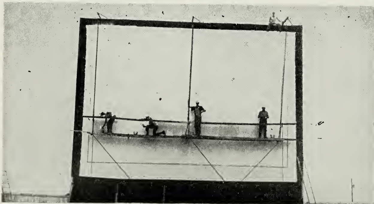
White's Drive-In, Nashville, North Carolina, recently equipped itself for the showing of 3-D films. A 40 by 30 foot canvas was used to cover the old screen. The canvas was waterproofed and then stretched tight. Workmen then applied coats of silver paint to supply required metallic surface.
